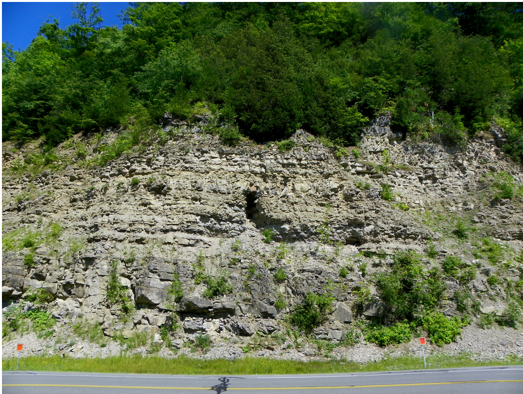
Figure 11 Chittenango Falls NY 13 Section: Massive beds at base are „Cobleskill” Formation with Chrysler dolostones above. Dark patches (excavations) are where collectors obtained Celestite crystals over the years. Arrow marks approximate position of the Silurian-Devonian boundary.
